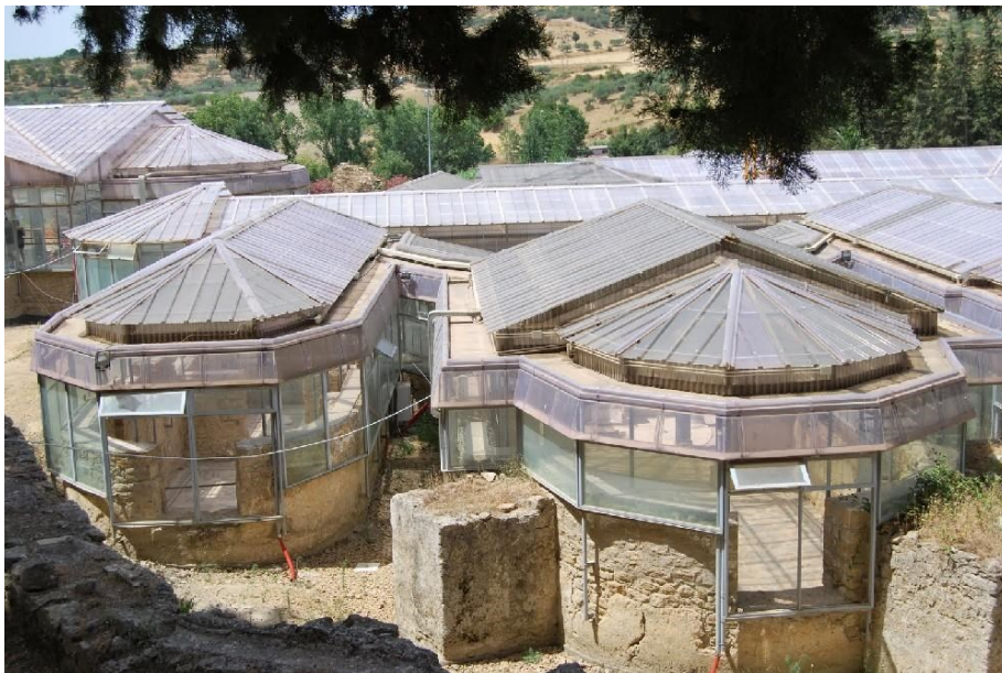
Figure 20 The shelter construction for protecting the mosaics.
