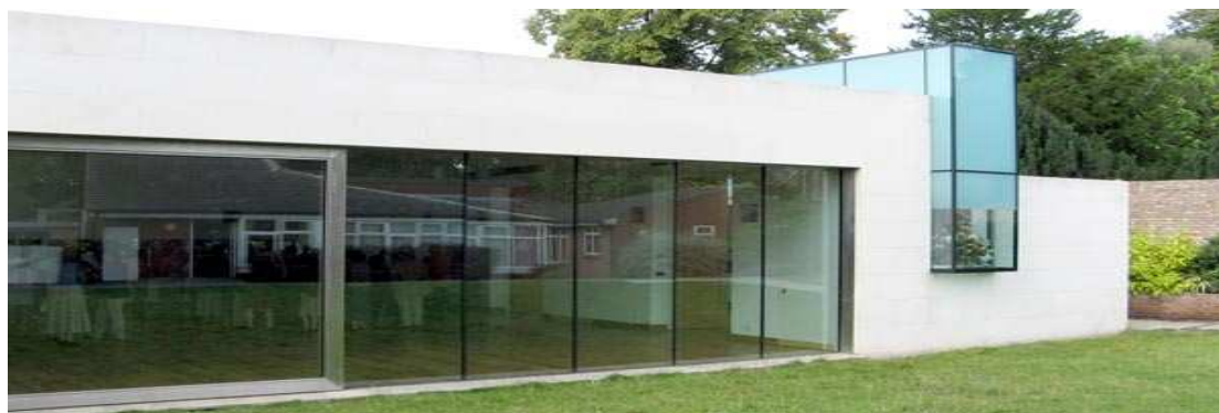
The Garden Hall built close to Anglican St. Mary's church in Wimbledon is a spacious, modern hall, with a lobby, kitchen and toilets for variety of function, both secular and religious. 315
