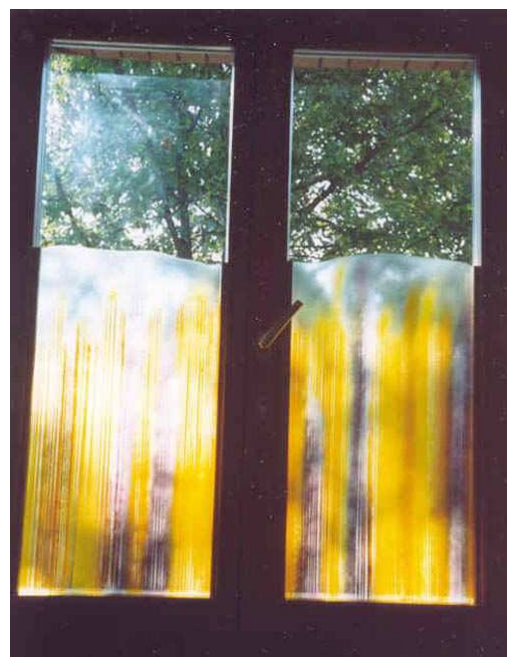
A sanded glass attached onto the window (M. Štědra).
