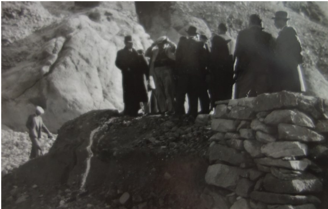
Fig. 1: Inspection of Czechoslovak experts at Saveh Dam, Iran, (1940s). Source: Archive of ČVUT, f. Theodor Ježdík, k. 71, 9/6/2/ Saveh (Írán).
